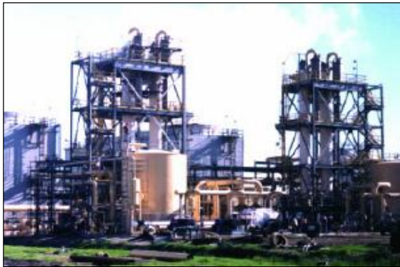
Figure 4: 4,600 m 2 self-cleaning heat exchanger surface replacing 24,000 m 2 conventional surface.
